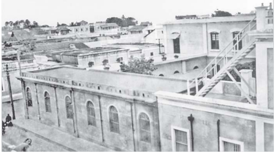
Cold Storage block
